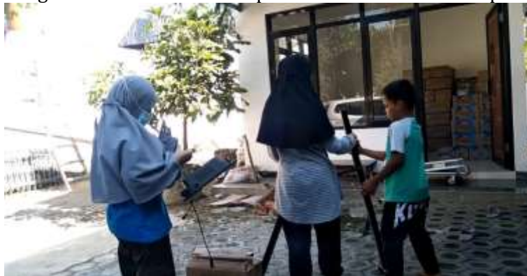
Figure 2. orphanage children helping in the installation of lights
