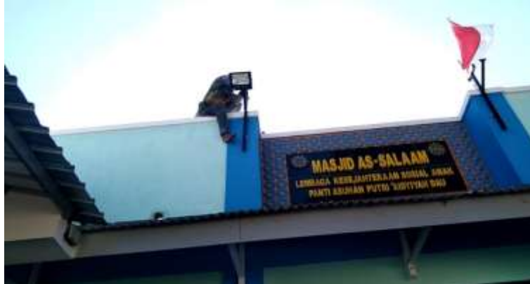
Figure 3. The team is installing solar chell lights at the Panti location
